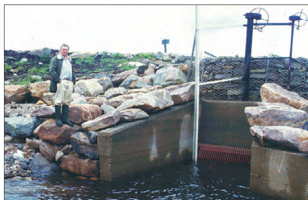
The intake weir for the Loch Garbhaig hydro scheme (J Butler)
