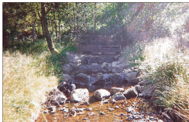
Concrete steps on Allt an Achaidh should be eased ( C Macdonald )
