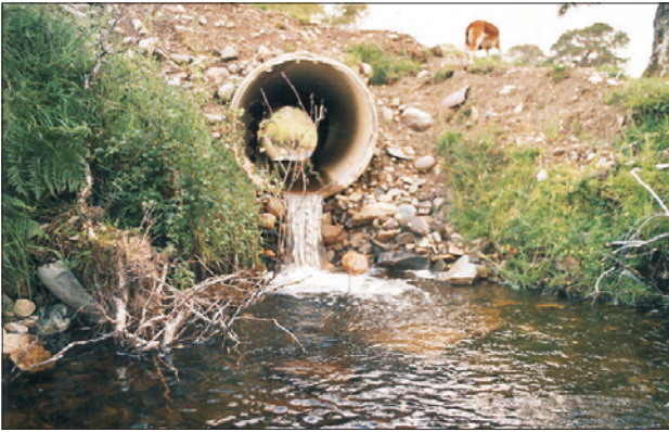
Culvert pipe on a tributary of Allt Doire Beithe, Coulin Estate (K Starr)
