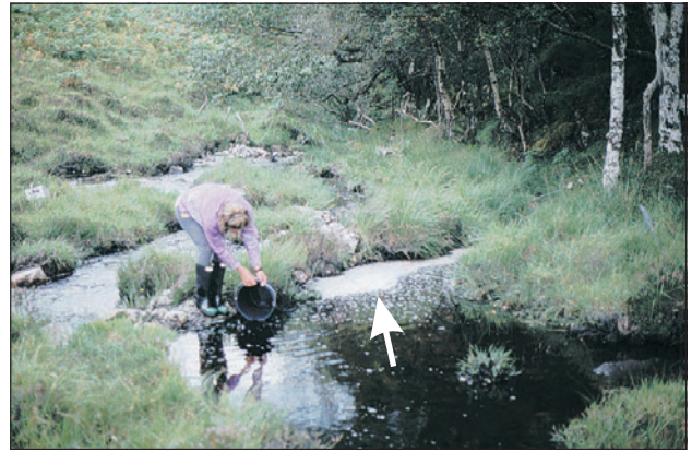
The inlet channels of the Allt Loch Ghiuragarstidh salmon ladder (arrowed) require renovation ( J Butler )
