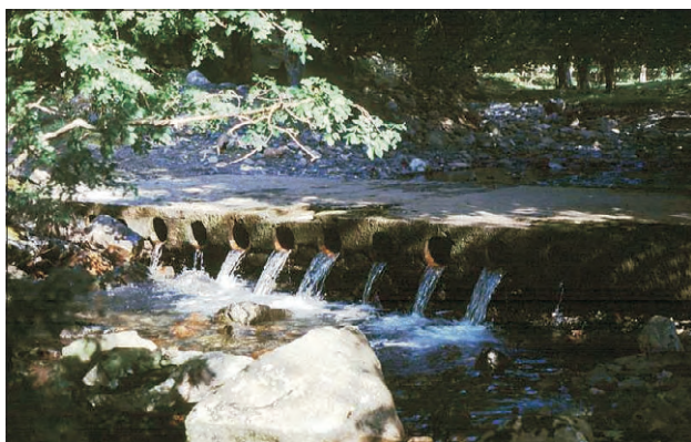
The Irish bridge on Allt Folais obstructs passage to a large area upstream ( J Butler )
