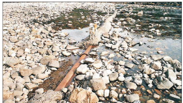
The Kinlochewe village septic tank outlet: further overflows into the Kinlochewe River must be prevented by Scottish Water ( K Starr )
