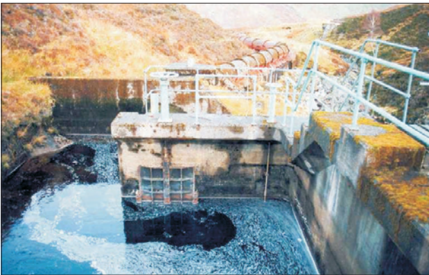
The intake of the Allt a Claiginn–Loch Fannich aqueduct (K Starr)
