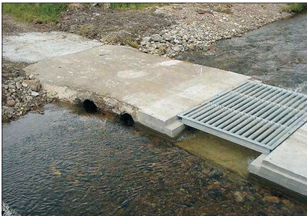
The Irish bridge on Allt Folais, Letterewe Estate, could be easily rectified, as in this example ( D Macdonald )
